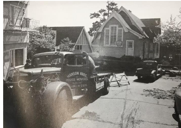
Truck and parish hall during moving process, 1954
